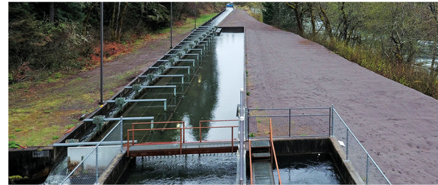
The Farmers Screen allows fast-moving water to pass through, carrying fish and debris back into the river, while a specialized weir lets slow-moving water fall into the irrigation canal, above . Below , water flows down a stream from the pass-through at Dead Point.
